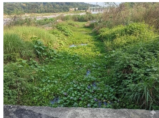
Image 7-9: Silting in the Kriya Ghat I&D Structure and overflow of grey water directly in the Kosi river
