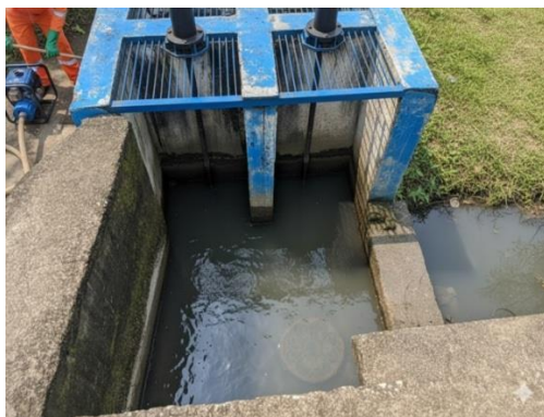
Image 7-9: Silting in the Kriya Ghat I&D Structure and overflow of grey water directly in the Kosi river
