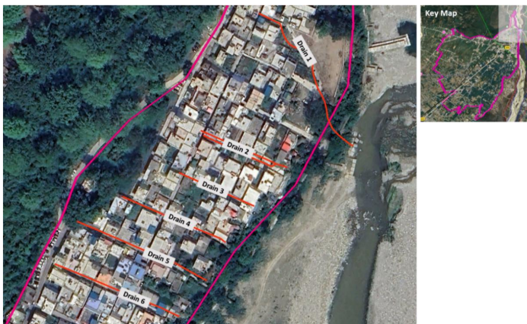
Image 4-6: Minor Drains directly fall into kosi river
