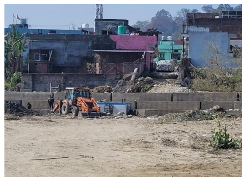
Image 3-10: Concrete Wall Near Ward 1
