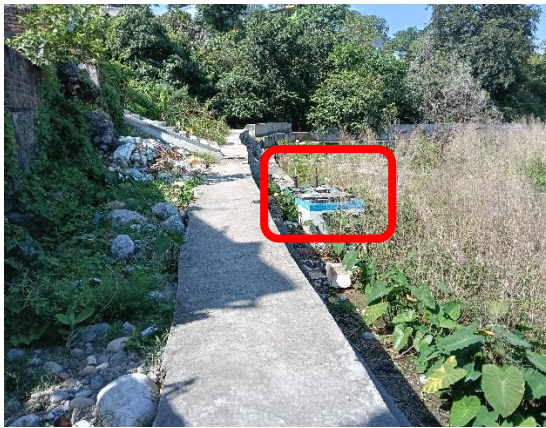
Image 7-3: Redundant of I&D at Pampapuri
