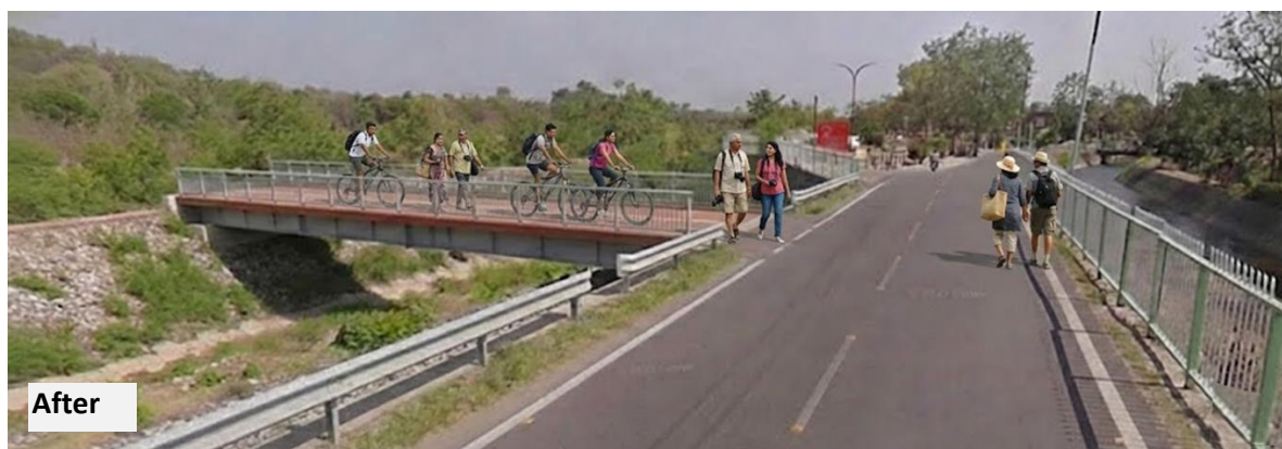
Image 7-20: Pedestrian bridge across the canal silt ejector channel
